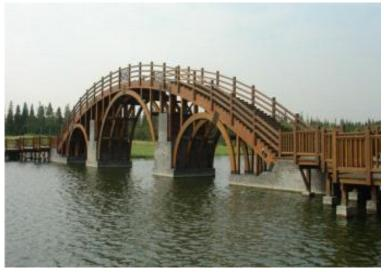
Timber is the oldest known bridge construction material. It can be used to build the most natural and beautiful structures. The Glulam Bridges are strong and economical. The Glulam bridges can last up to 100 years when properly pressure treated and maintained.
