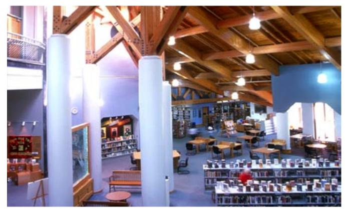
Components made of glulam are easily worked and produced using energy-efficient and environmentalfriendly manufacturing processes that offer excellent opportunity to customize both shapes and sizes.
